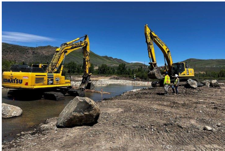
Work on the Colorado River Connectivity Channel progressed throughout 2023.
