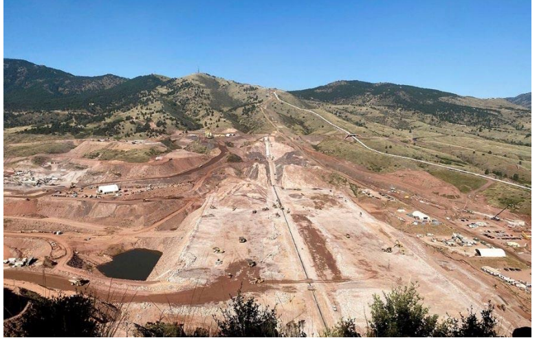
Construction on the Chimney Hollow Reservoir made great strides in 2023.
